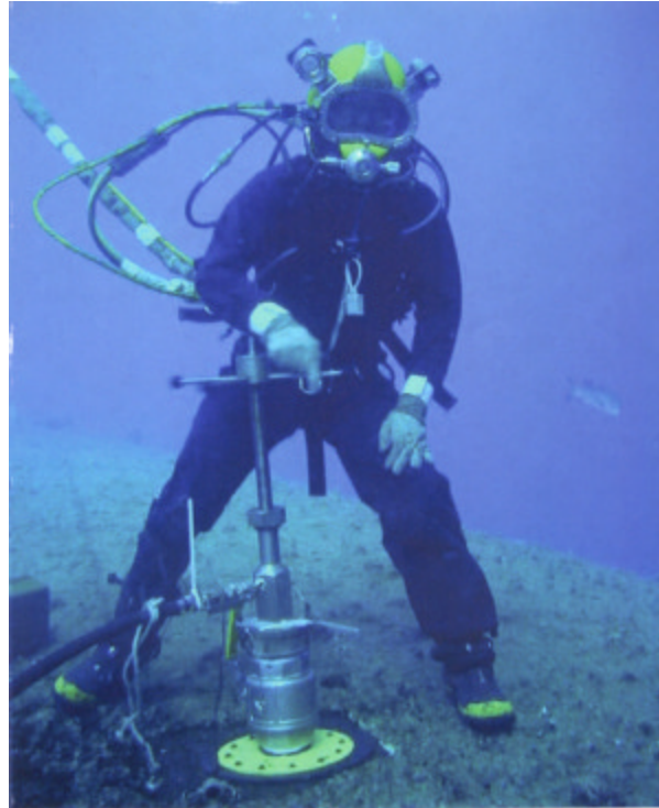
Figure 8. Lightweight hot-tap.
